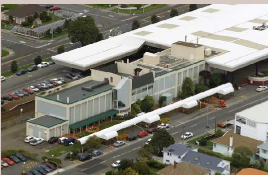
Waterloo Water Treatment Plant
