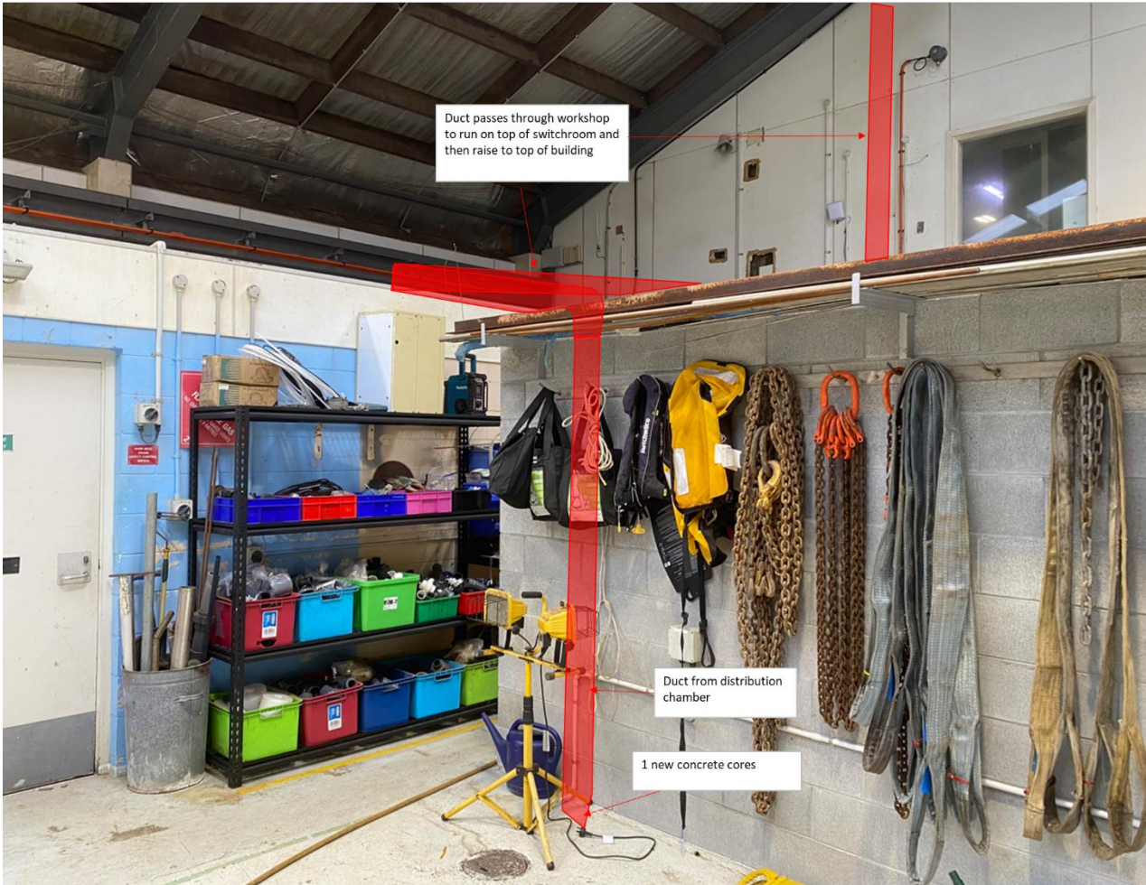
Figure 3-20: Option 2b (AC, BTF and BTF+AC) Duct from distribution chamber travels to top of peaked roof
