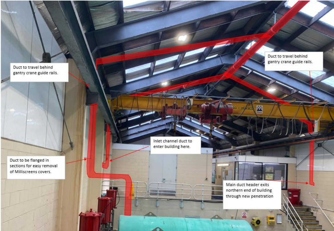
Figure 3-21: Option 2b (AC, BTF and BTF+AC) Milliscreens ductwork (only one shown) and main duct header.
