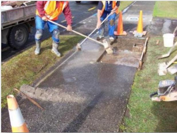
A good solution is to divert the slurry into the area cut as demonstrated above
