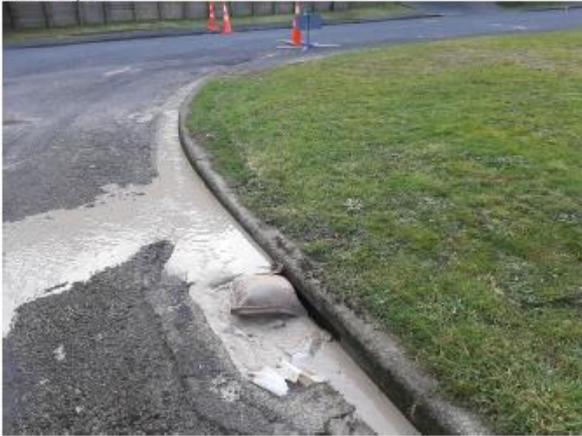
Filter cloth (bidim - Geotextiles) that I have seen on sites and are pictured above should not be used in drains/sumps as they do not filter sediment nor concrete slurry, the only possible use would be if you wanted to overlay the sump (including the sides of the sump) with several layers of bidim so nothing enters the sump to transfer the discharge from site to another sump further along the road, in which you may have a jet vac operating.
