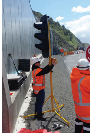
When ready to be used, loosen the lock screw and rotate the unit to face oncoming traffic
