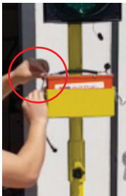
Lock latches to secure battery box
