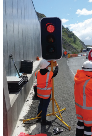
Once facing oncoming traffic, tighten locking screw
