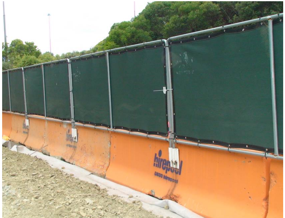
Visibility screens are to be used to help prevent motorists being distracted by the works to facilitate improved and safer traffic conditions.
