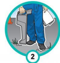
2 Use cable locating devices
