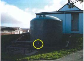
Note: Sample tap handle has been removed to stop tap being turned on when not needed. Tap handle required when taking samples.
