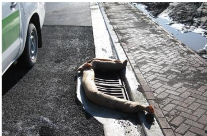
Pic 3. Filter socks for use controlling sediment and concrete slurry
