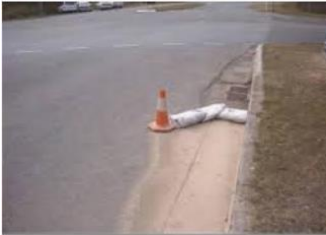
Pic 2. Sediment and concrete slurry controlling dams
