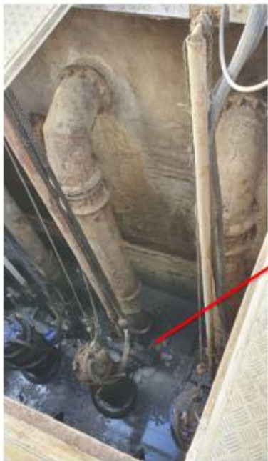
Leaking Pump Discharge Manifold
