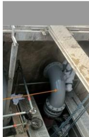
Leaking Pump Discharge Manifold
