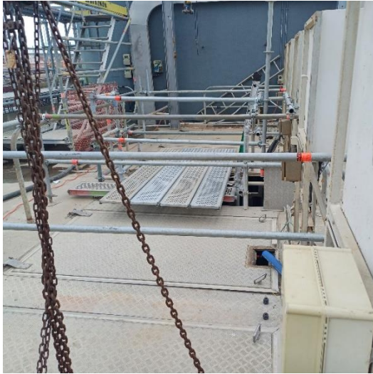
■ Figure 3: Moa Pt IPS Wet Well Access Scaffolding, 23 November 2024
