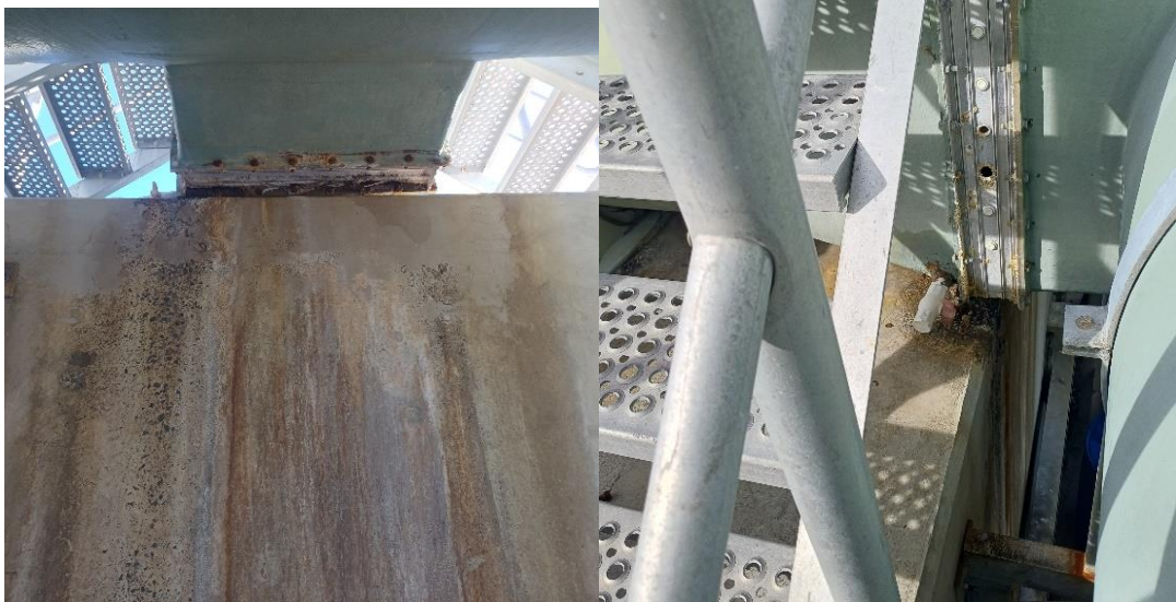
■ Figure 13: MBBR Flow Control Baffle, 23 November 2024
