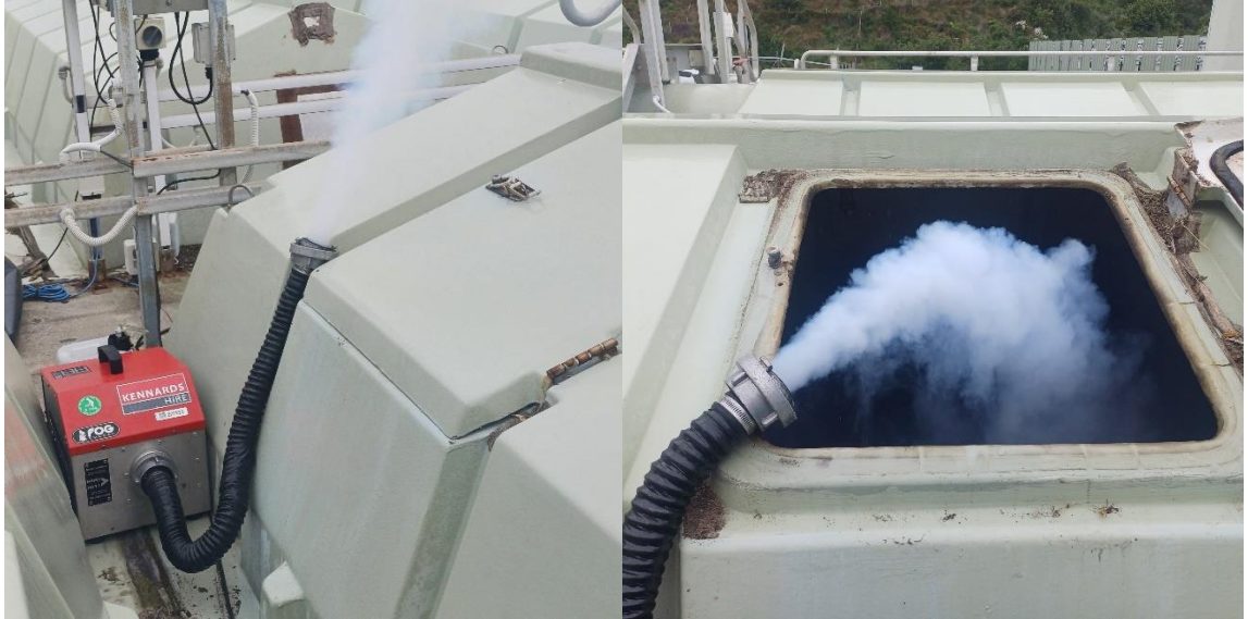
■ Figure 15: MBBR Tanks Smoke Test, 23 November 2024
