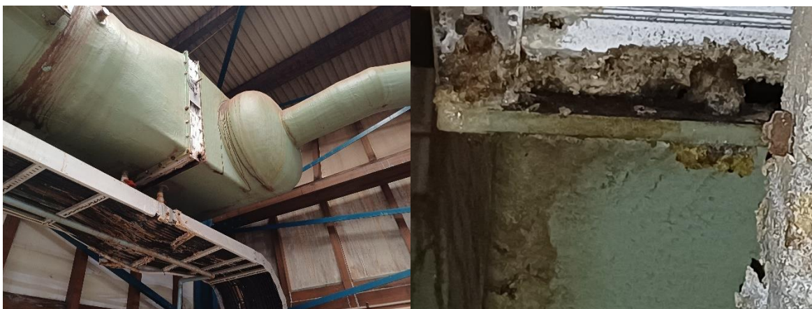
■ Figure 5: Primary Treatment Room Baffle, 23 November 2024
