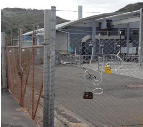
■ Figure 1: Site 1 Monitoring Equipment
