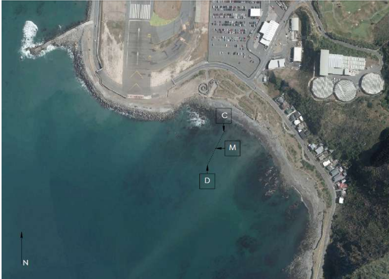
Figure 3: Shallow Water Section – Exposed Pipeline between positions C & D
