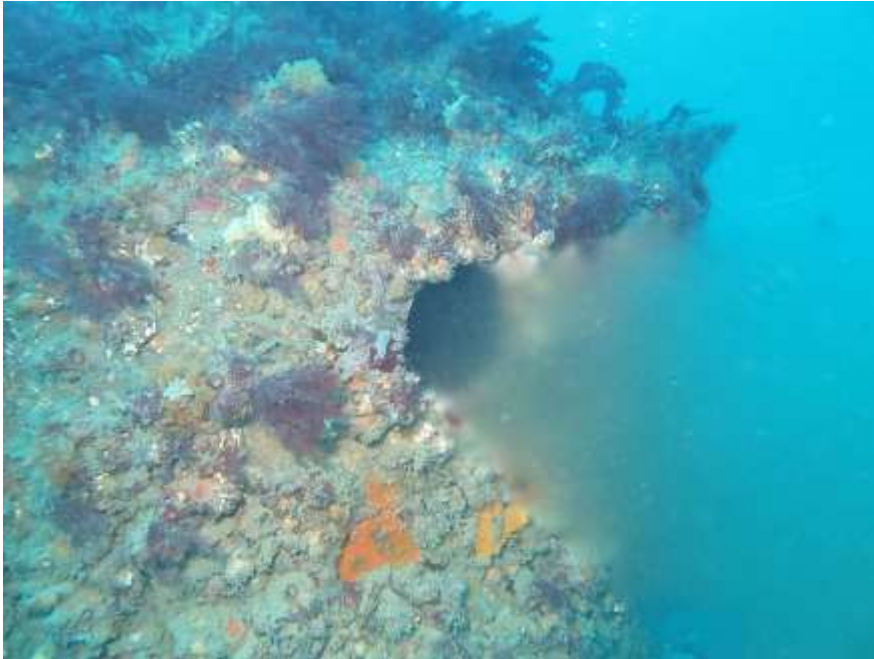
Figures 17 & 18: Diffusers in operation
