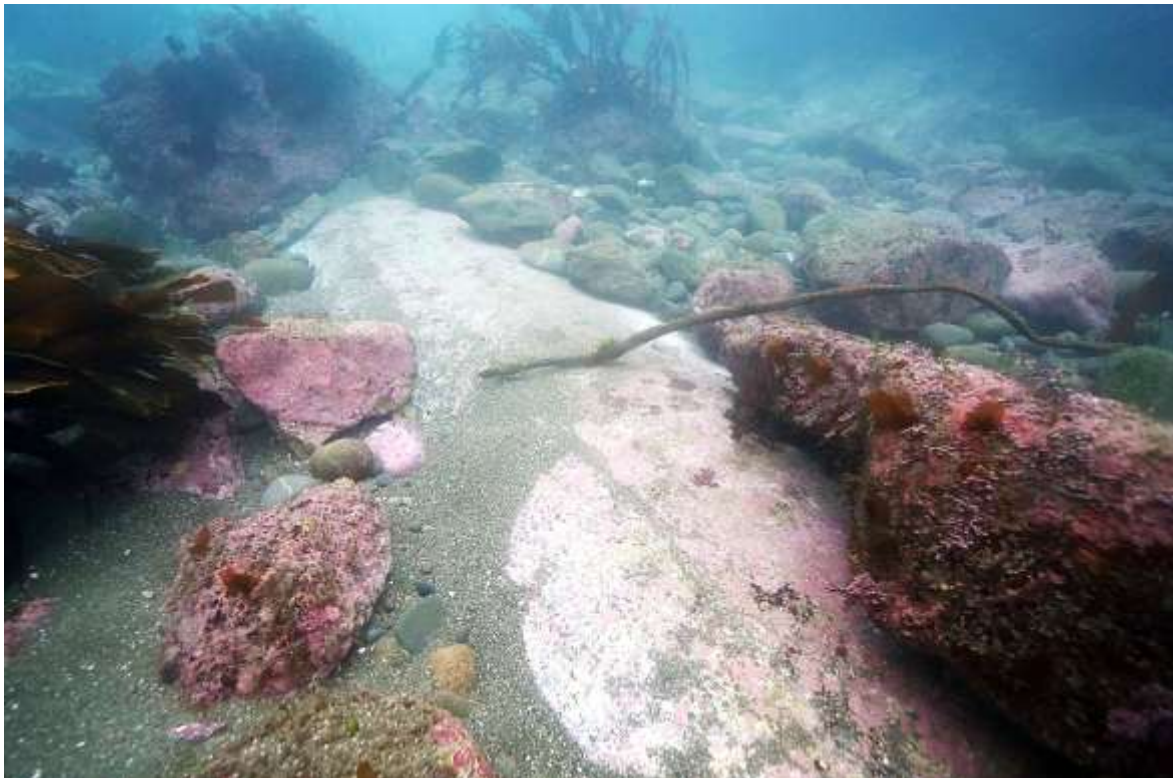
Figure 4: Zone C – shoreward position at which pipe exposure commences
