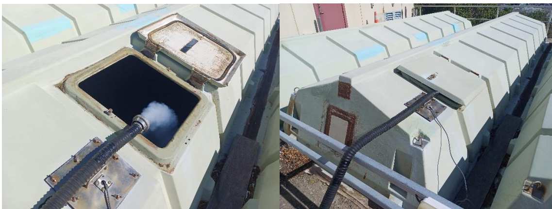
■ Figure 6: Moa Pt MBBR Tanks Smoke Test, 26 January 2024
