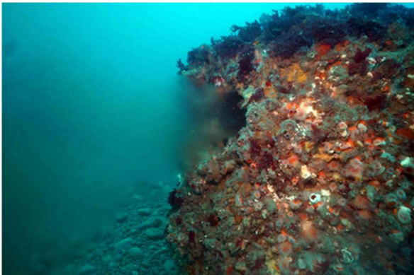
Plate 5: View of a diffuser riser and fouling assemblage, Feb 2021
