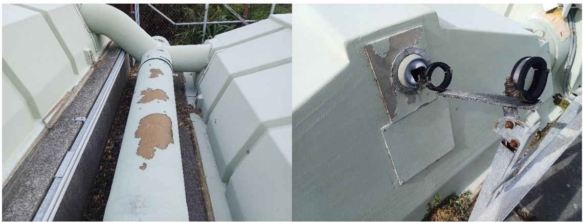
■ Figure 9: Secondary Treatment Enclosure Weather Paint and Holes, 26 January 2024
