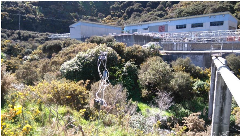
■ Figure 2: WTP Monitoring Site 2
