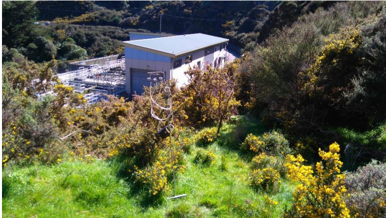
■ Figure 1: WTP Monitoring Site 1
