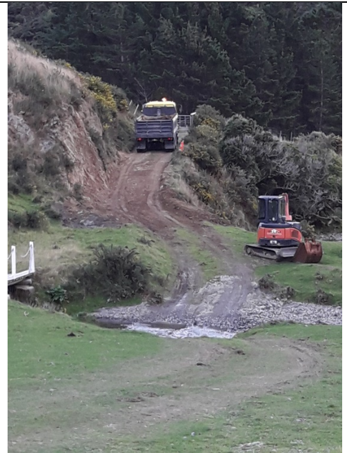
Constructed stream crossing at ch4550 to enable boulder delivery to ch4730.
