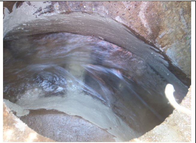
Photo of patching in manhole, post works, at ch4220.
