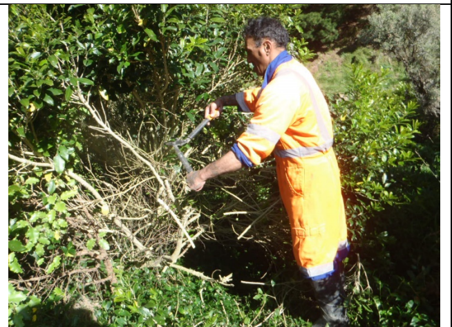
Photo of typical vegetation clearance around outfall pipeline.
