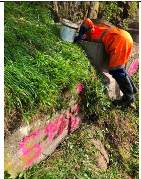
Photo of patching inside manholes ch5945 and ch5950s.
