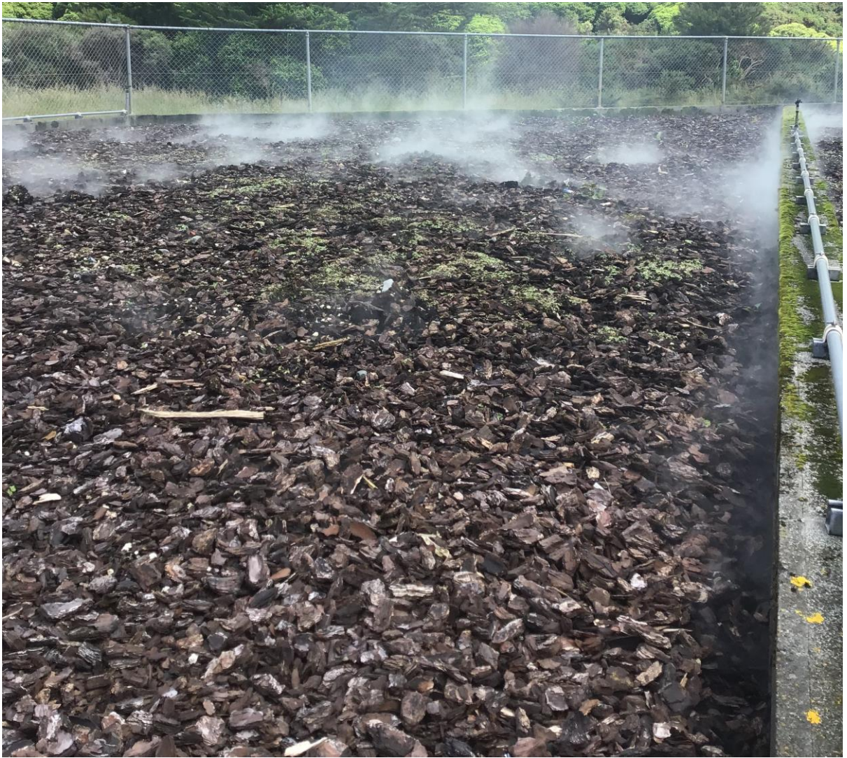
Figure 7 Cell 1 smoke test
