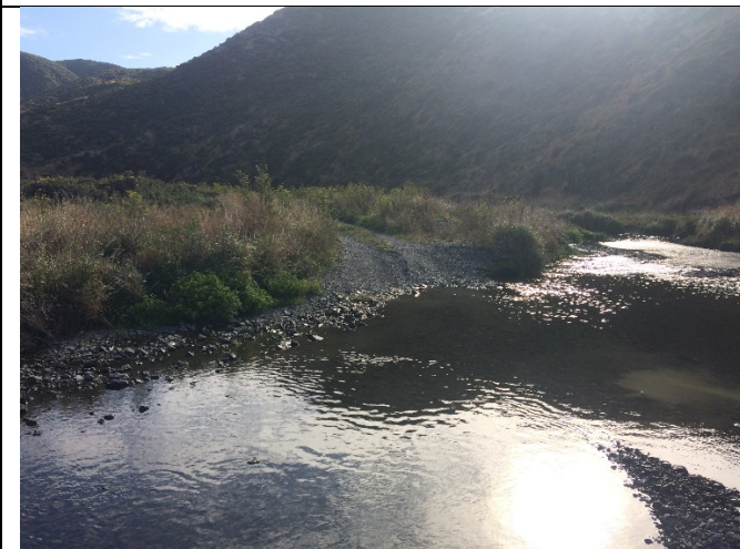
Photo of formed stream crossing at ch925.
