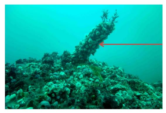
Figure 23: Diffuser # 1 (seaward southern- most diffuser) - CP test point. Readings at this position provide evidence of electrical continuity through the diffuser section
