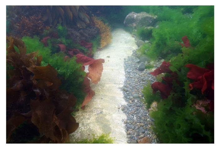
Figure 3: Shoreward of the 00.0 metres monitoring mark, a further 03.0 metres of pipeline has been exposed
