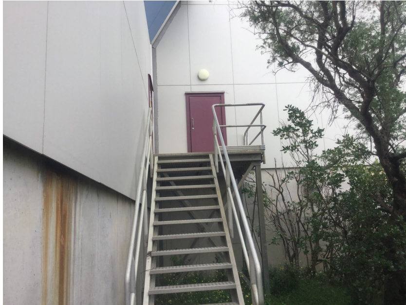
The other door into the Primary tank
