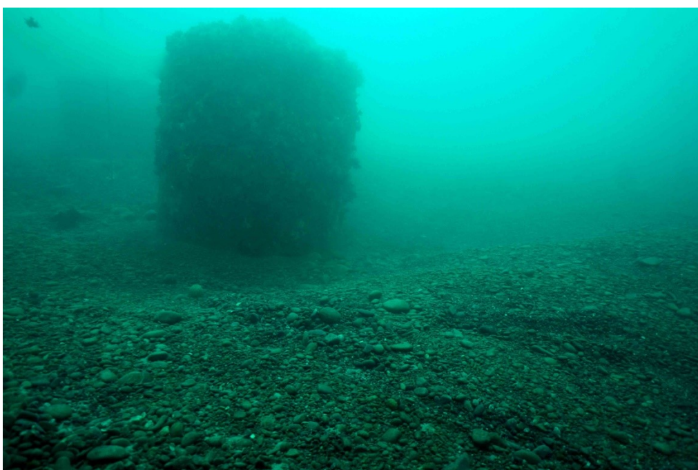
Figures 18 & 19: At diffusers where greatest scour depths were measured, examination was completed for any evidence of exposed erosion control mats; however no sighting of any such material was made
