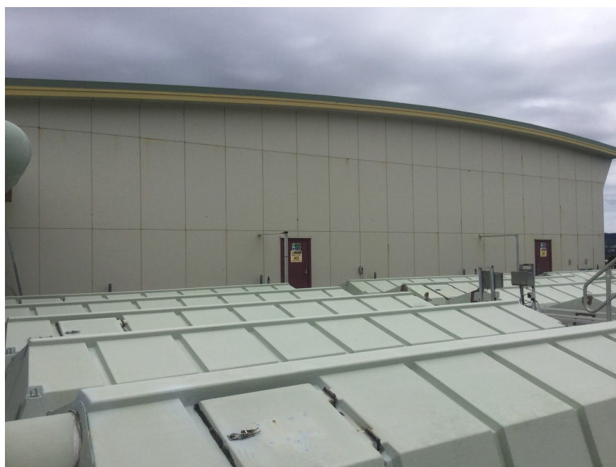
Primary Tank Roof looking west
