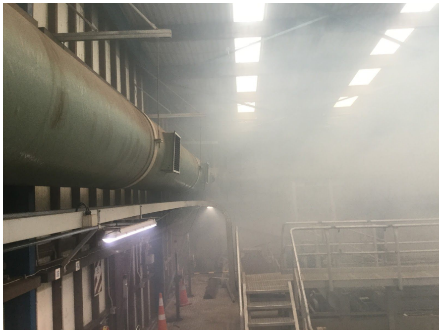
Smoke being drawn into the extract grills
