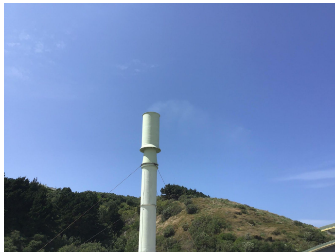
Smoke discharging from Moa Point stack
