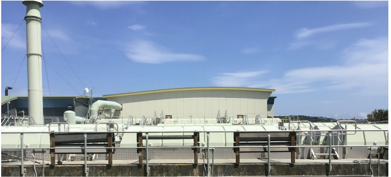
Primary Tank Roof looking West
