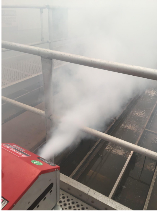
Smoke machine starting to saturate the Primary Tank area
