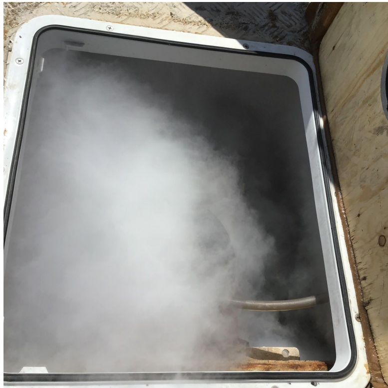
Smoke inside sample hatch
