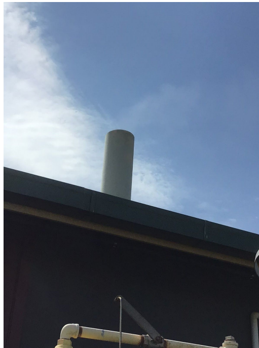
Smoke discharging from the IPS stack
