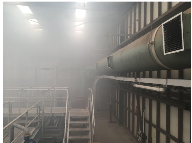
Smoke being drawn into the extract grills
