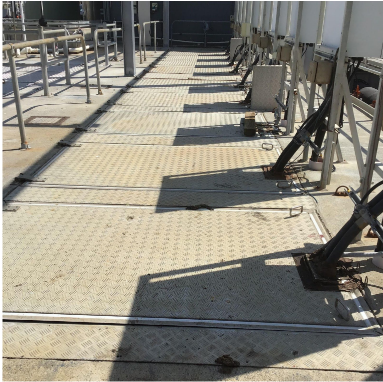
IPS Pump Hatches
