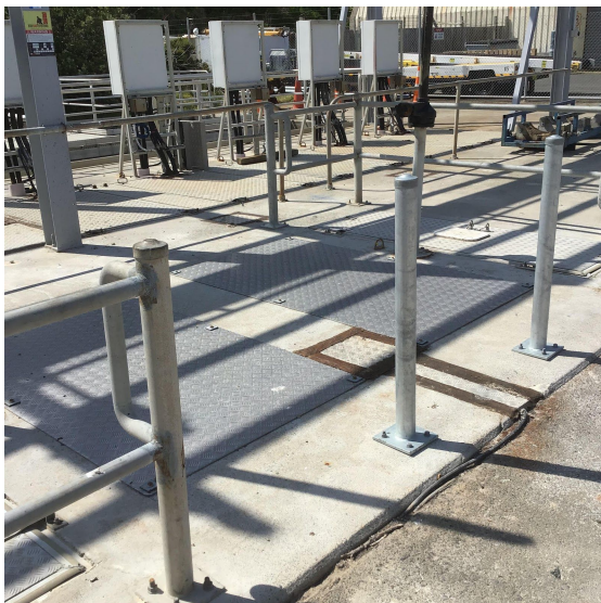
Sealing tape around hatches
