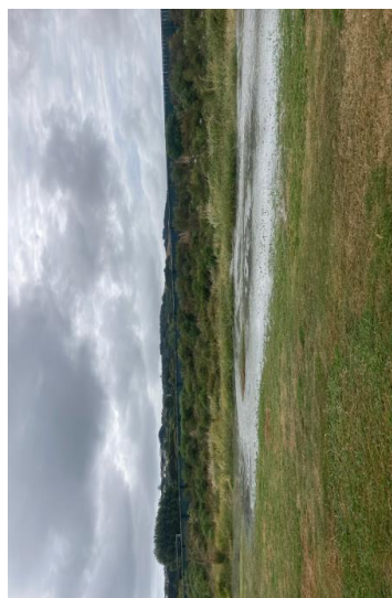
Site of the burst drinking water pipe which feeds into the Plimmerton Reservoir
