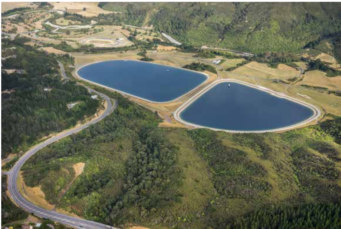
The Macaskill water storage lakes in Te Marua, Upper Hutt, Wellington's largest water storage facility
