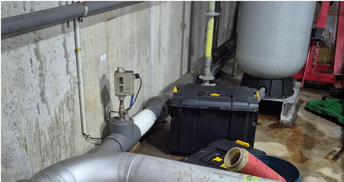
Figure 32: RE Pressure switch
