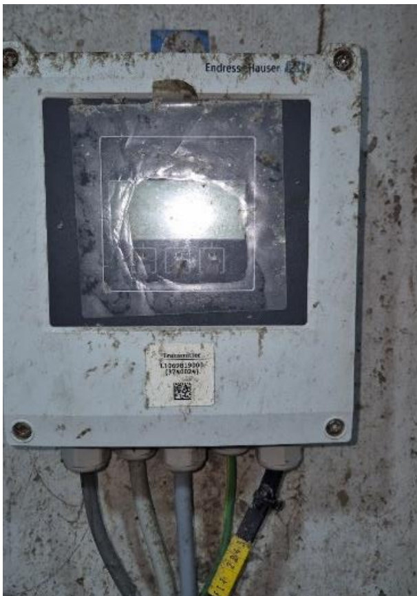
Figure 26: Primary sludge flow transmitter (L) and PLC remote IO cabinet and power supply for flow meter (R)
