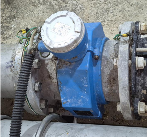
Figure 37: Flow meter (L) and transmitter (R)
