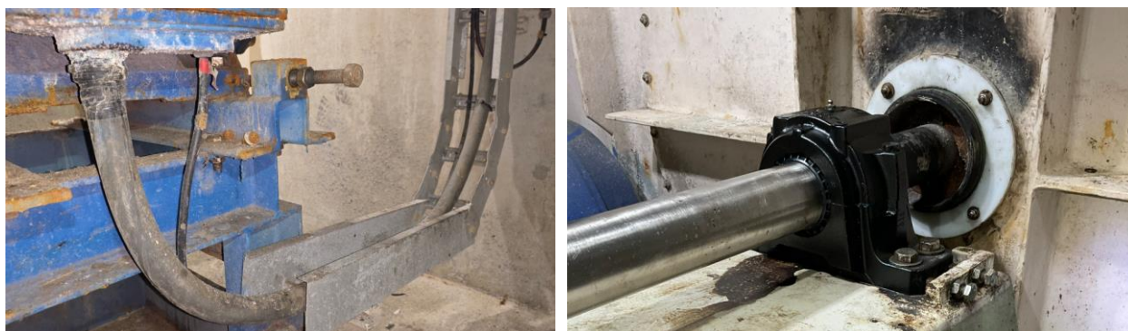
Figure 11: Scrubber Extraction Fan Motor Cables and Terminal Box (L) and Scrubber Extraction Fan 2 Bearing (R)
