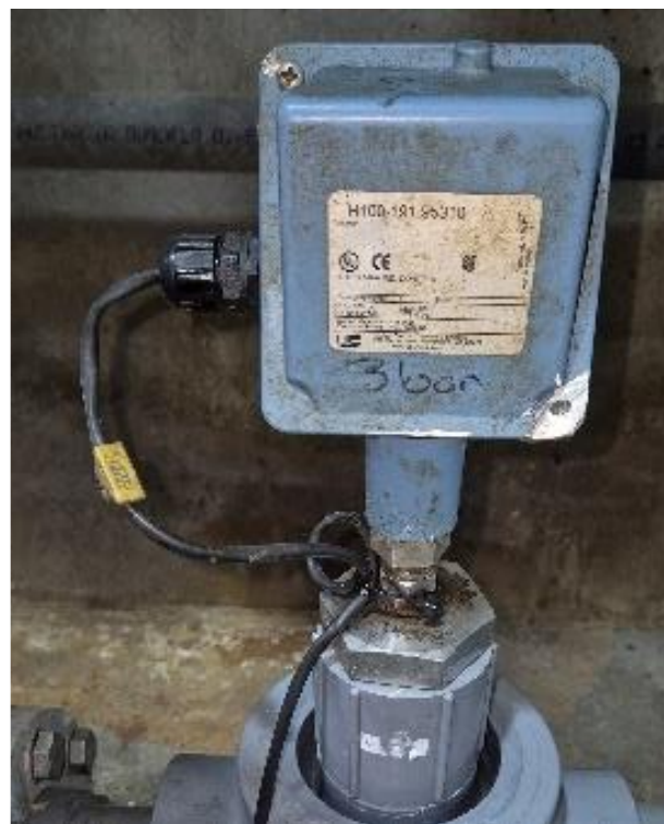
Figure 29: Primary sludge pump termination boxes (L). Pressure switches (R)
