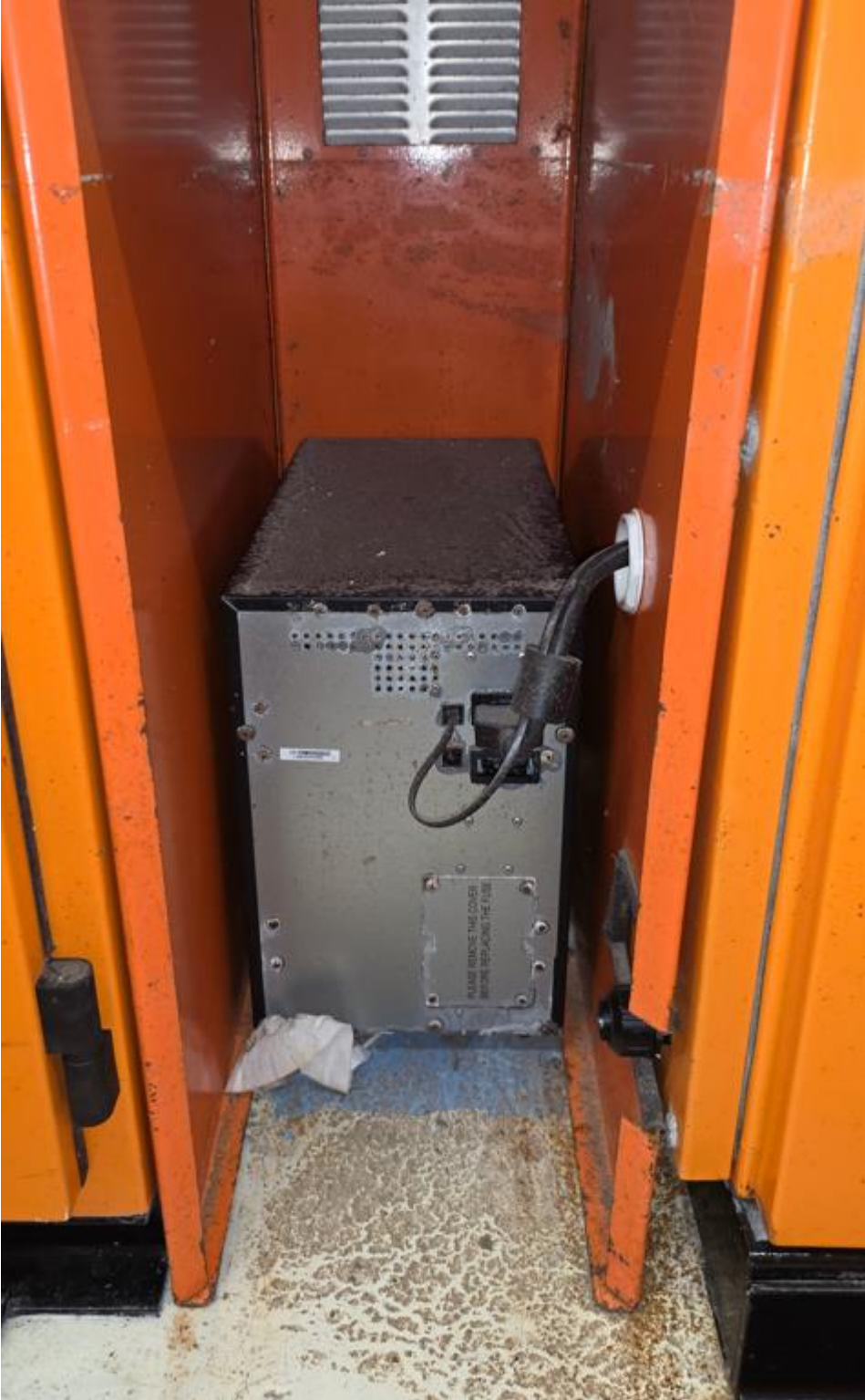
Figure 82: Fully submerged power supply
