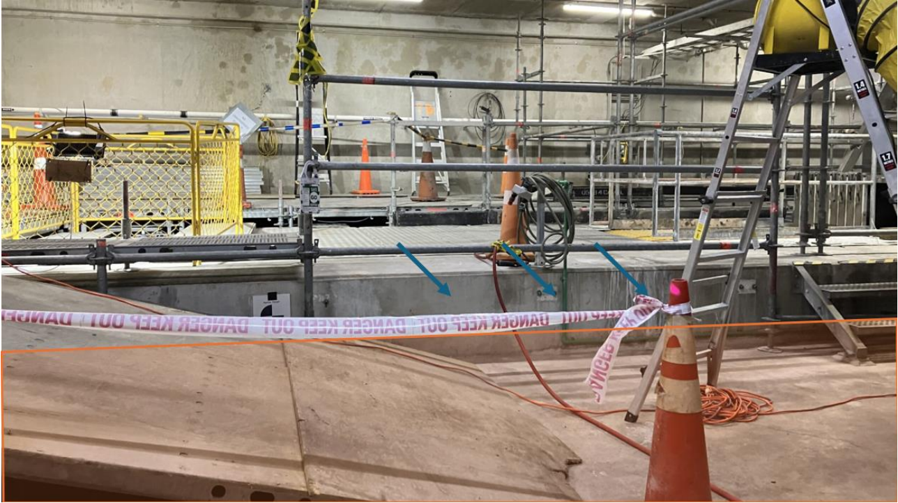
Figure 90: UV Room indication of the approximate level to which assets were submerged
