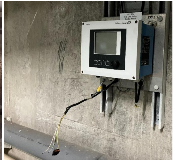
Figure 55: Top: 3x RAS and 1x WAS Flow Transmitters on Panel, Bottom Left: WAS flowmeter, Bottom Right: RAS Sludge Density Transmitter (not in service).
