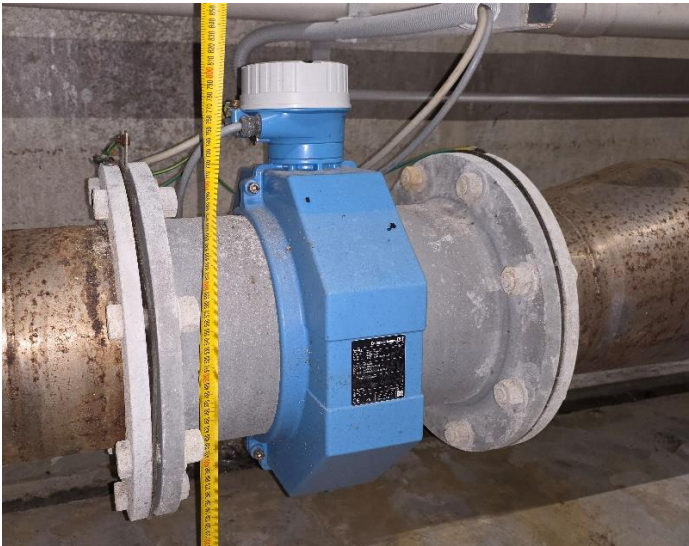
Figure 55: Top: 3x RAS and 1x WAS Flow Transmitters on Panel, Bottom Left: WAS flowmeter, Bottom Right: RAS Sludge Density Transmitter (not in service).
