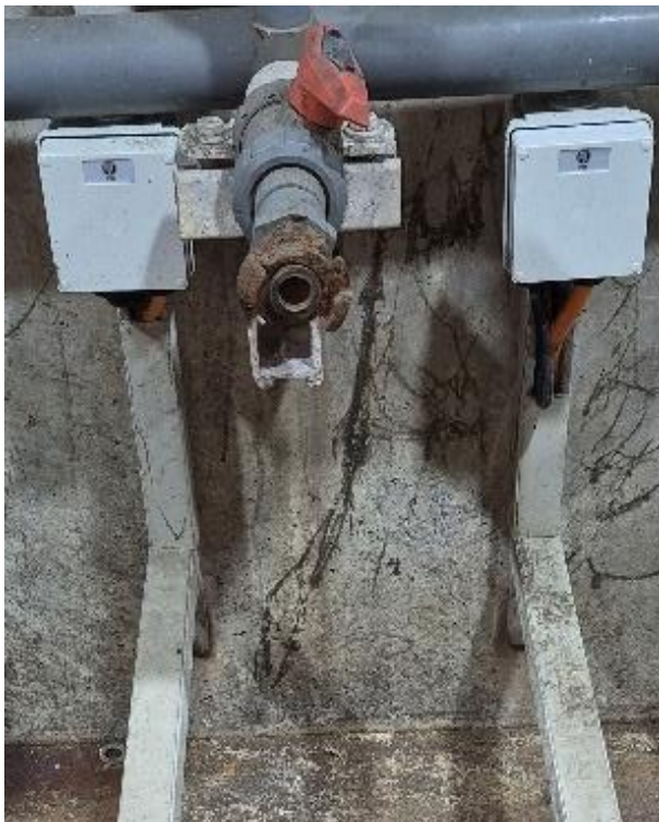
Figure 29: Primary sludge pump termination boxes (L). Pressure switches (R)
