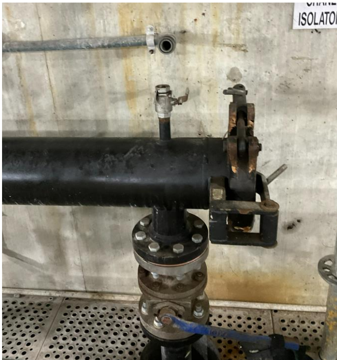
Figure 46: Sludge transport pig launcher arrangement
