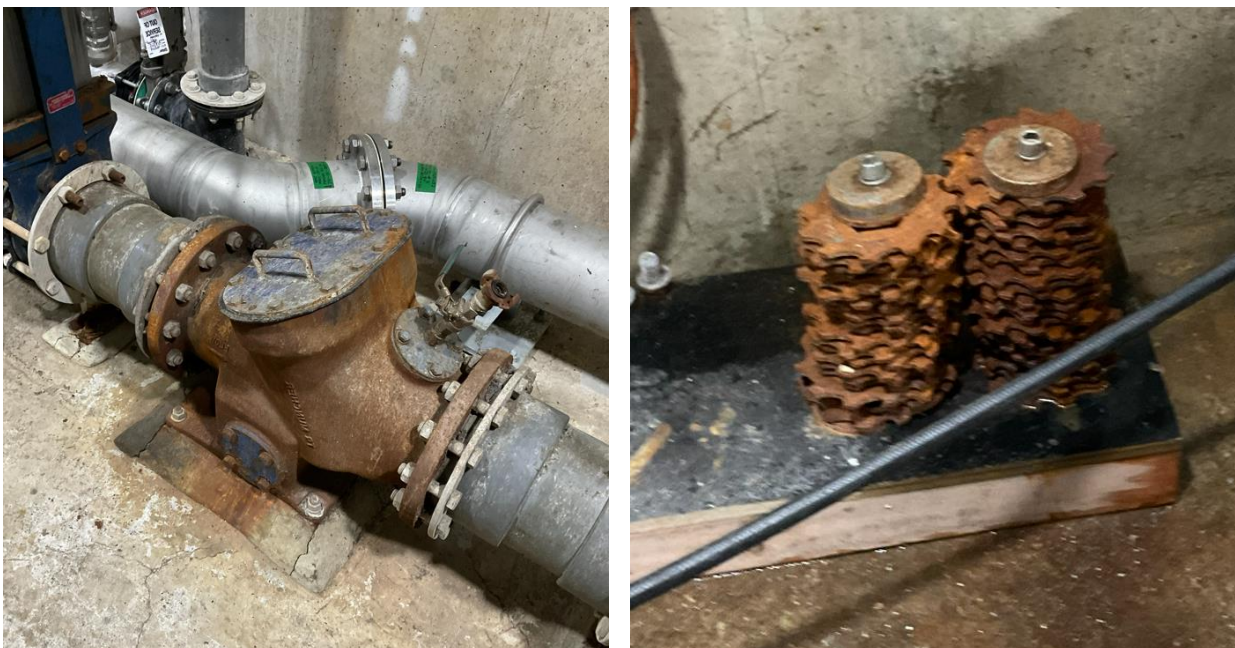
Figure 38: Muncher without motor installed (L) and Muncher cutters (R)
