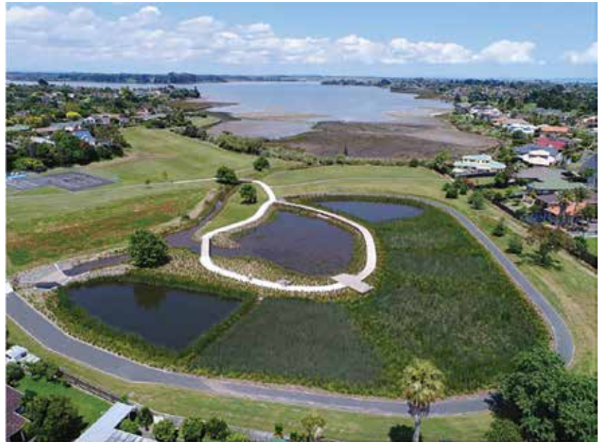
Brylee Reserve, Auckland: A recently completed constructed wetland integrated with a public park and houses.
