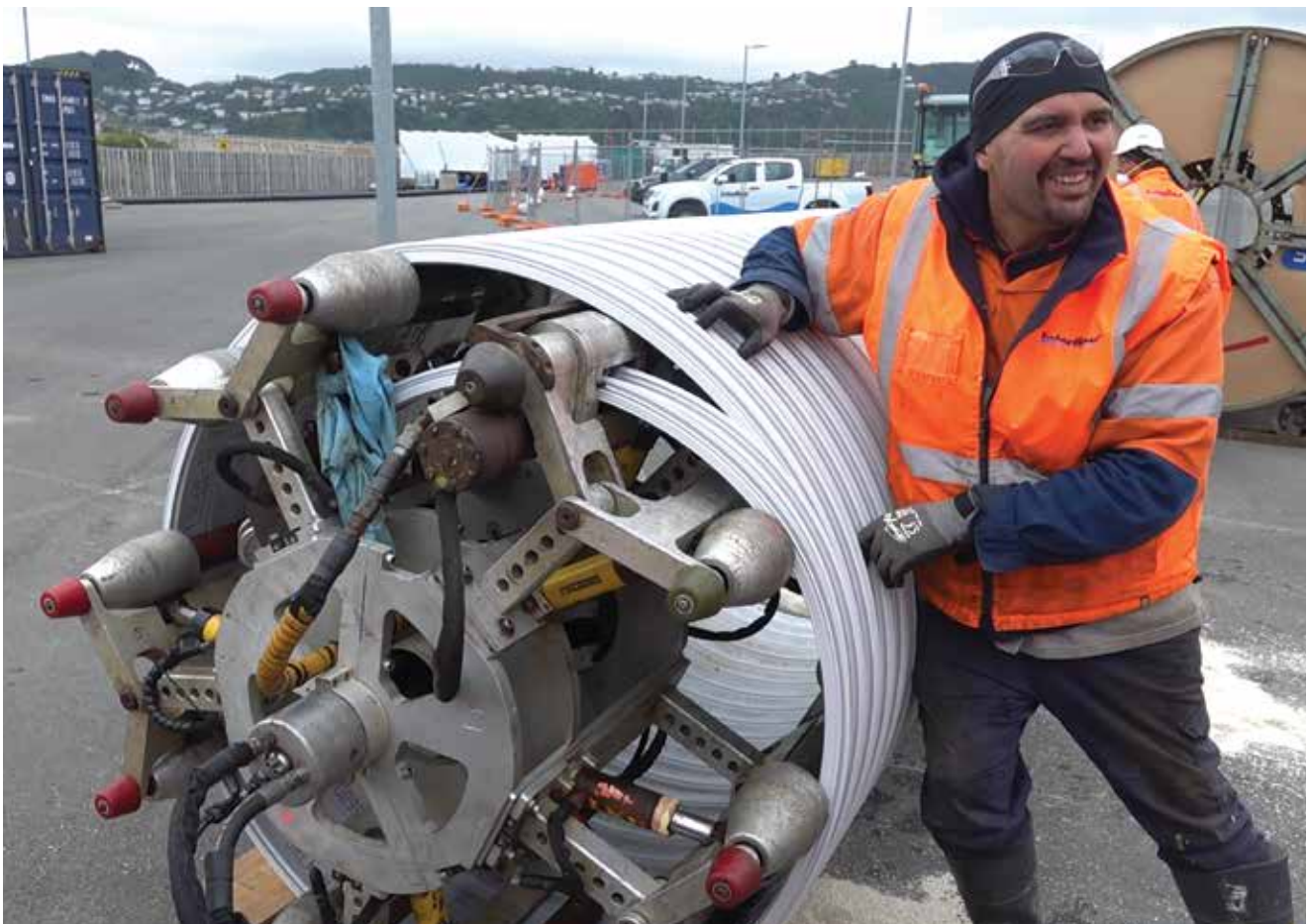
An above-ground demonstration of the pipe lining machine by Adam, a foreman for our contractor, Interflow, showed how the plastic compound spirals forward and is glued into place as it advances through the host pipe.
