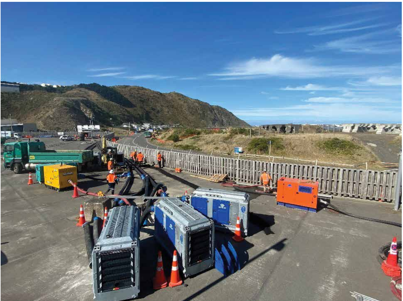
Pumps and temporary piping were used to by-pass the corroded section of pipe.
