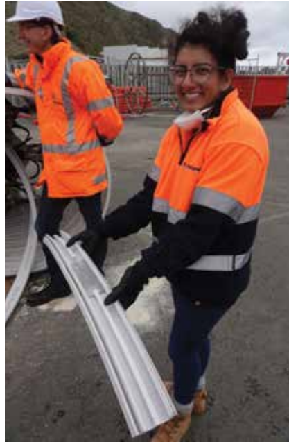
A durable, long-term solution: Saadia Ali with a section of the PVC used to line the interceptor.
