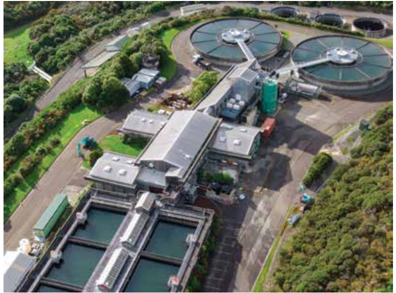
Te Marua Water Treatment Plant typically treats around 60 million litres of water daily.
