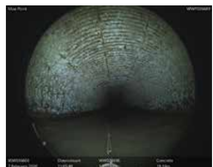
A CCTV view of the interceptor's reinforced concrete interior revealed corrosion caused by hydrogen sulphide.
