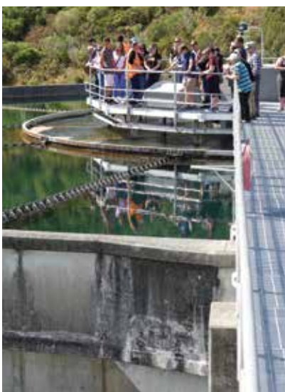
Production from Te Marua accounts for just over 40 per cent of Wellington Water’s supply in a typical year.
