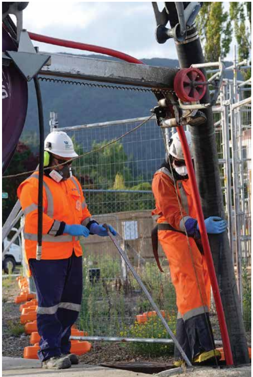
We created strict safety guidelines for our crews and provided them with the personal protective equipment they needed to stay safe while doing essential work during lockdown.
