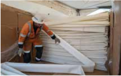
The 1.8km-long liner was manufactured in Germany and shipped here under urgency for the repair during the Covid-19 Level 4 lockdown.
