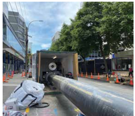
Sections of the temporary pipe situated above ground on Willis Street were welded together on site.
