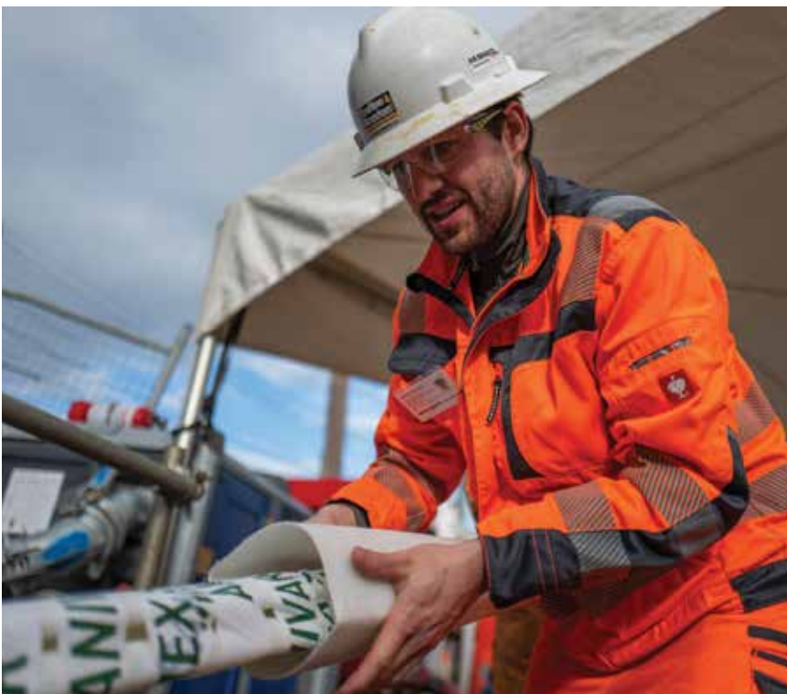
The pandemic delayed the manufacture and installation of the liners made in Germany to repair the Mt Albert sludge pipes.
