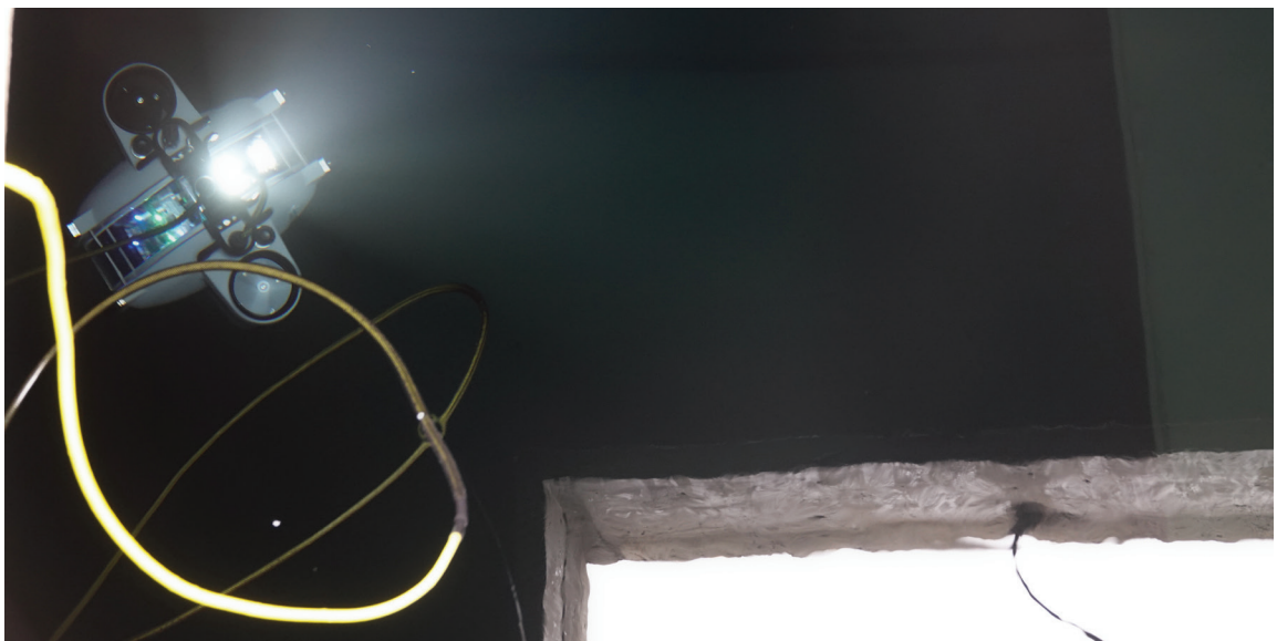
The underwater ROV about to dive on a reservoir inspection. A 100m signal cable is needed for the largest tank reservoirs.
