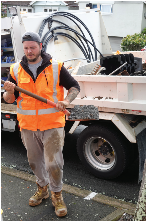
Wet earth is taken away and replaced with dry gravel.
