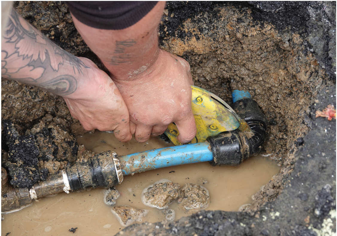
Cutting the leaky elbow connector for removal.
