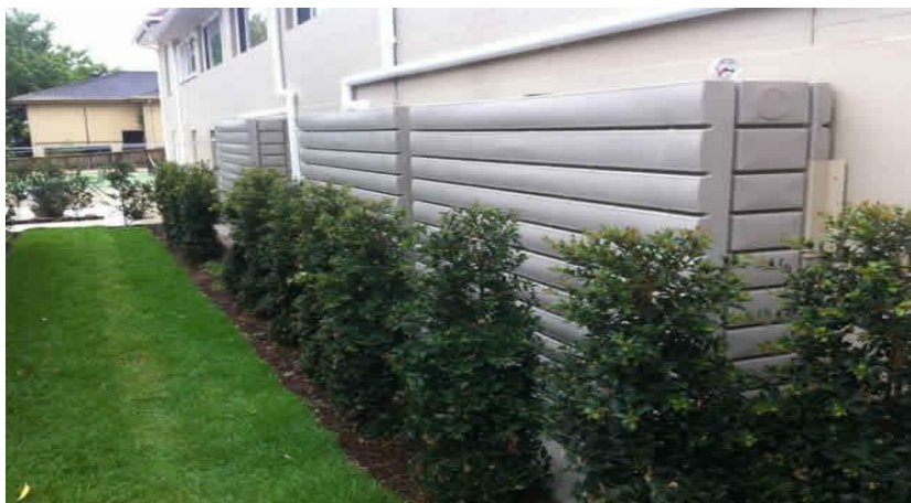
Storage tanks to achieve hydraulic neutrality
