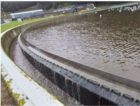
Image 5: Clarifier 1 - At Capacity
