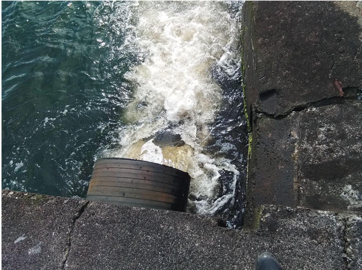
Photo 1: Rukutane Outfall – Dated 27 September 2023
