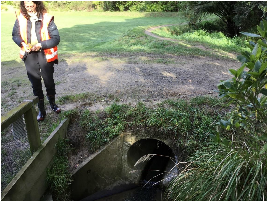
Figure 6b – Culverted crossing. Culvert interior dimension 690mm. Bund visible top centre.
