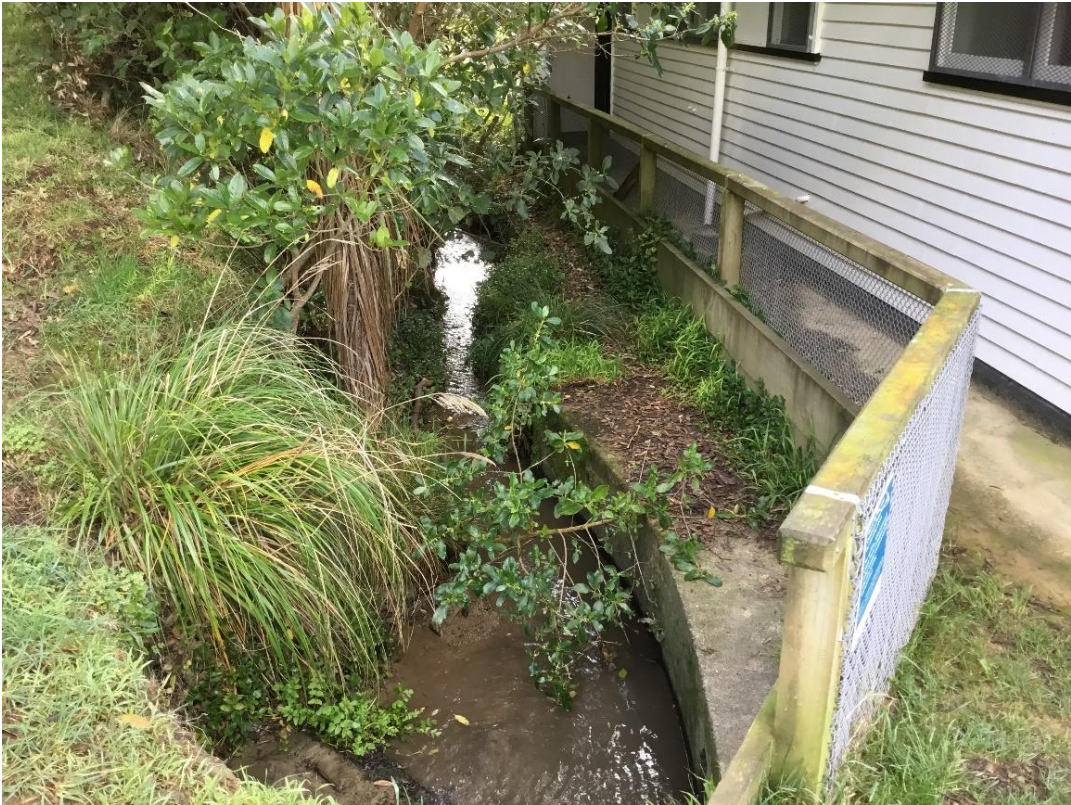
Figure 6c – Sports pavilion with Papawai stream descending along its eastern wall.
