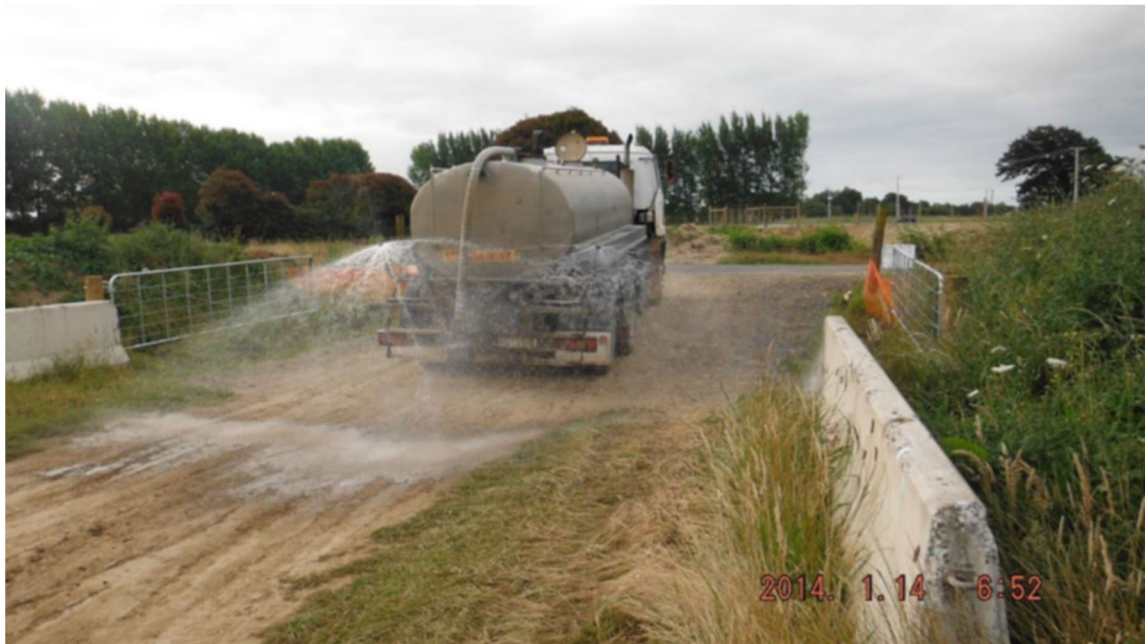
Photo 7: Water Cart in operation
