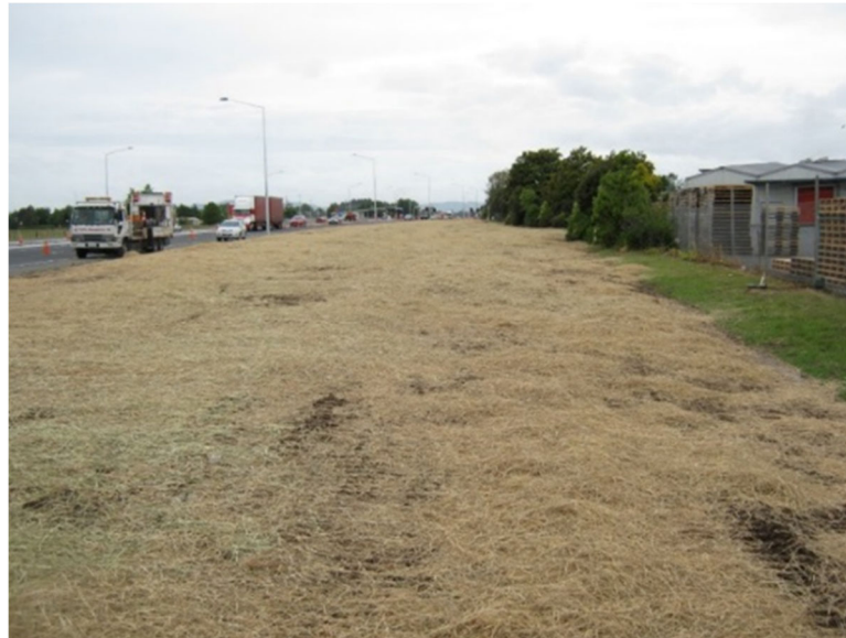
Photo 3: Hay Mulch applied to large surfaces following completion to stabilise.
