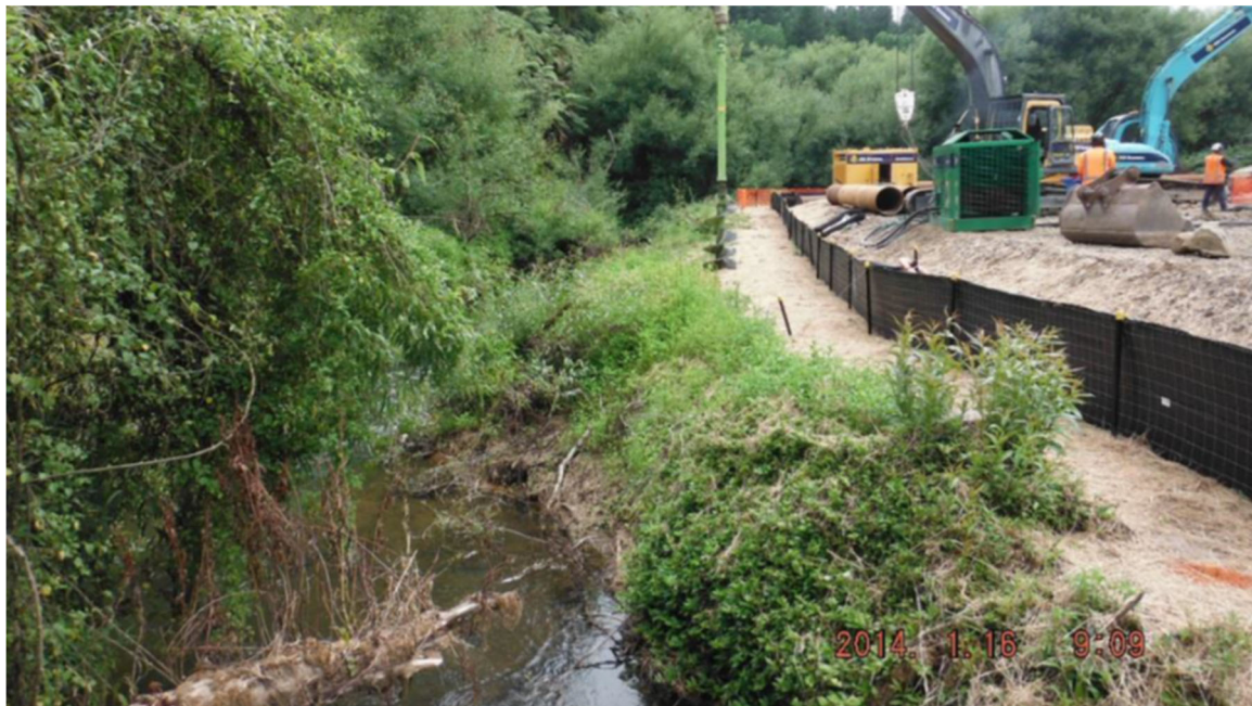
Photo 4: Super Silt Fence
