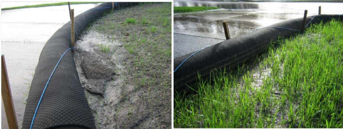
Photo 1 & 2: Silt or Filter Socks used as edge protection.
