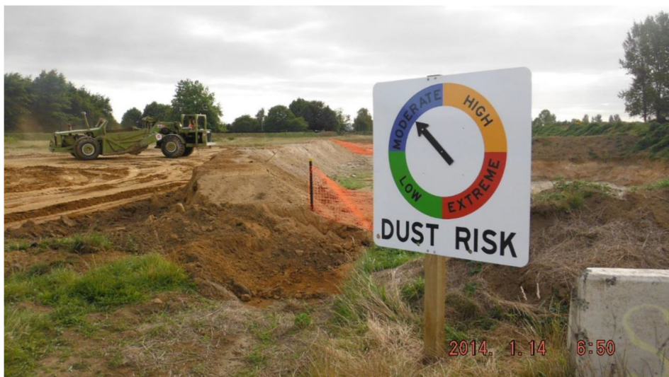
Photo 8: Dust risk signs will assist with communicating the risk to construction staff.
