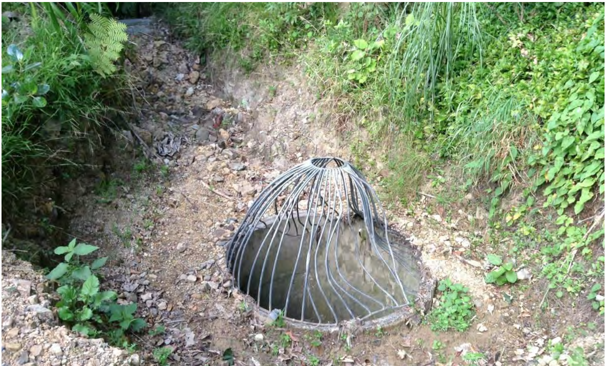
Photo 28: The scruffy dome at the bottom of Papawai Stream. The stream can be heard beneath the deep gravels which were deposited during flooding in May 2015.
