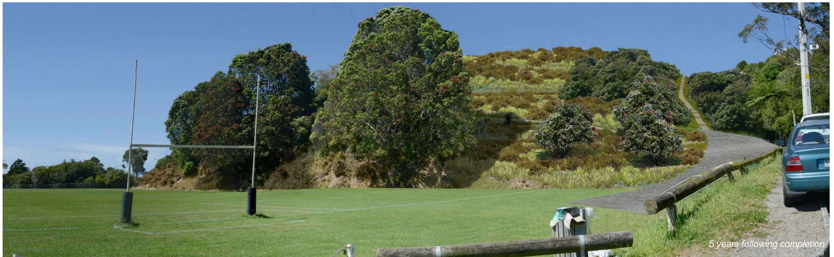
View during construction
