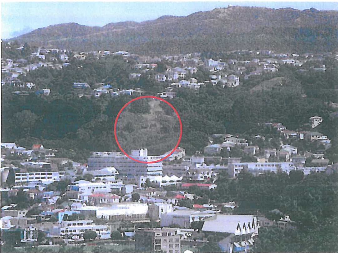
Figure 5-1: View of Prince of Wales site from the east
