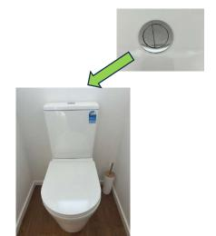
A **half-flush** button makes the toilet use less water to flush.
