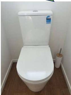
A **half-flush** button makes the toilet use less water to flush.
