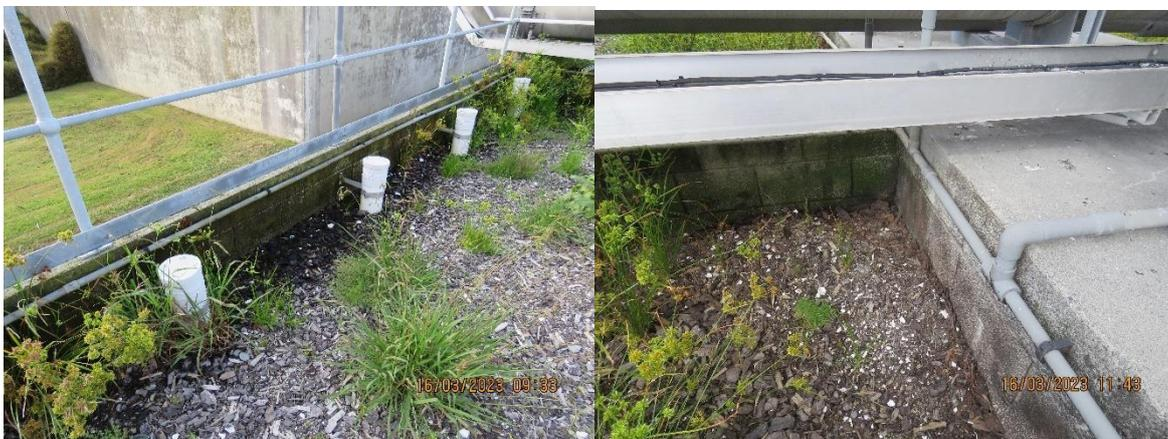
■ **Figure 4: Biofilter Dry Spots and Short Circuiting, 16 March 2023**
